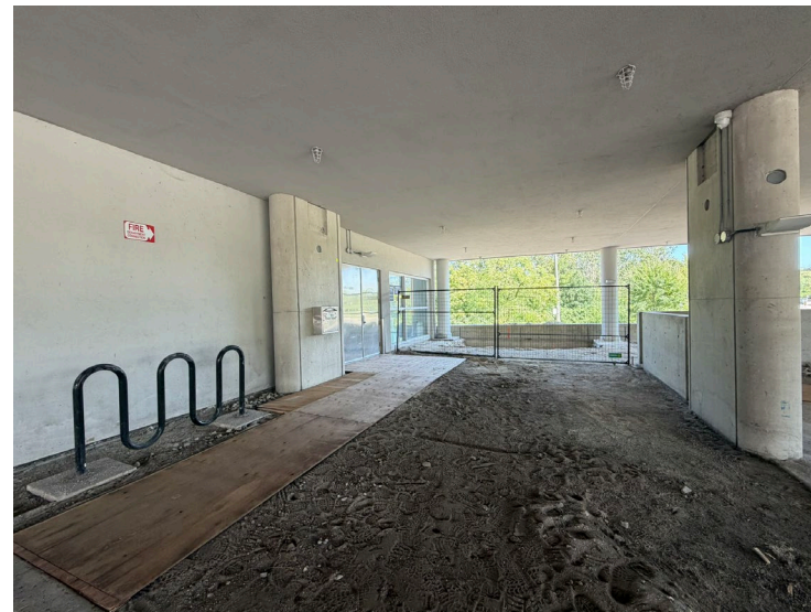
Paving removed at front entry
