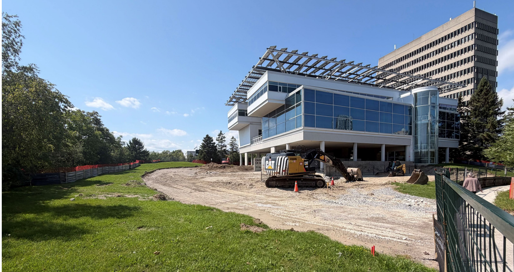
View from Moatfield Drive of ongoing construction – late August 2026
