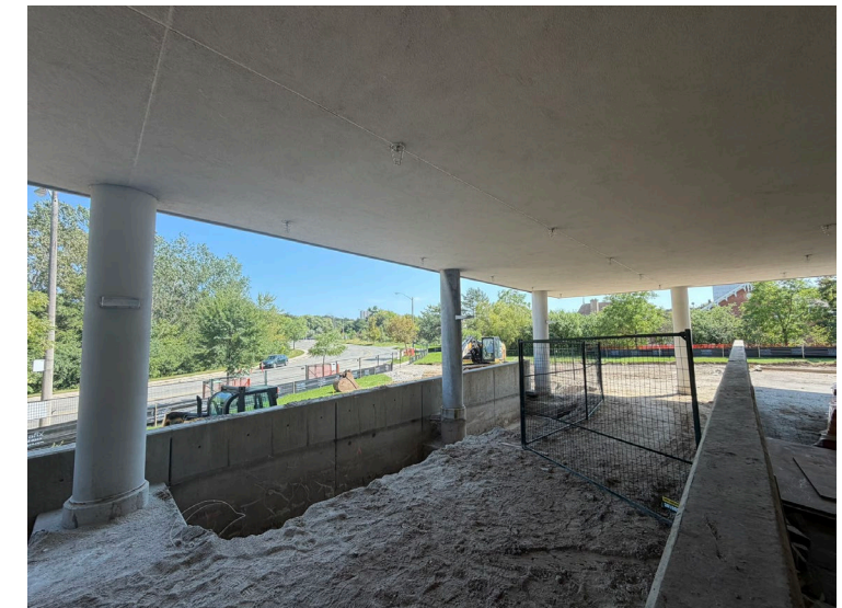
Pedestrian paving removed – pier foundations exposed
