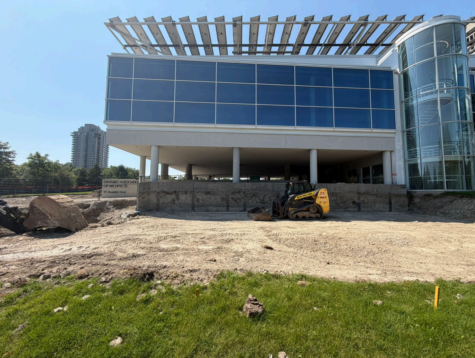
View from Moatfield Exposure of concrete retaining wall to be removed
