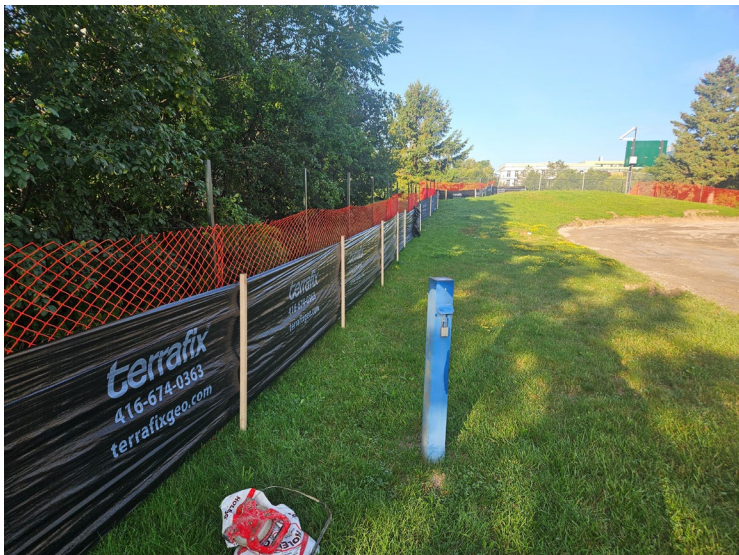
Silt & Tree Fencing south of driveway – Monitoring Well
