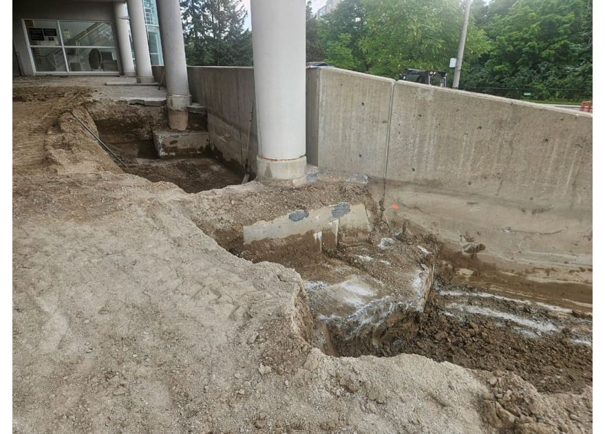
Building column pier foundations exposed
