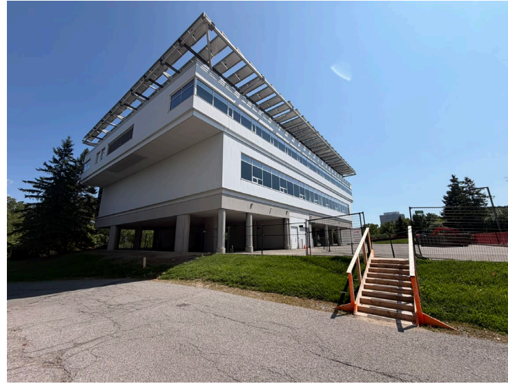
Temporary Pedestrian Stair Entry from North Driveway
