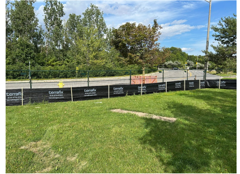
Perimeter / Silt Fencing along Moatfield Dr. frontage
