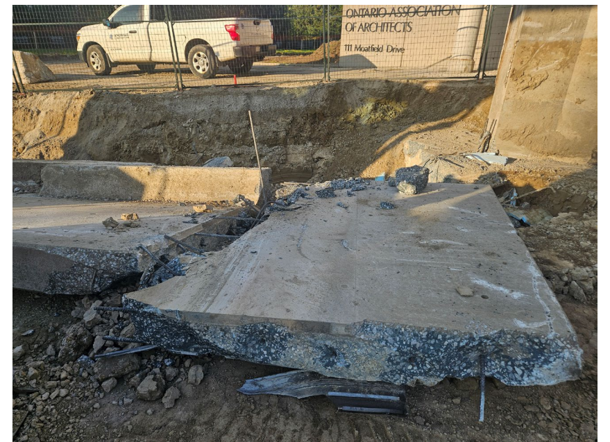
Portion of existing concrete wall removed
