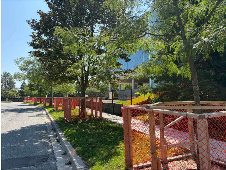
Tree Protection fencing along Moatfield
